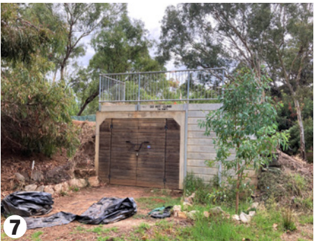
7 Culvert storage under berm with raised viewing platform over.
