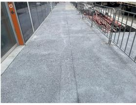
Works are continuing on the Eastern side of Pitt Street with the first section of exposed concrete footpath being placed in February.
