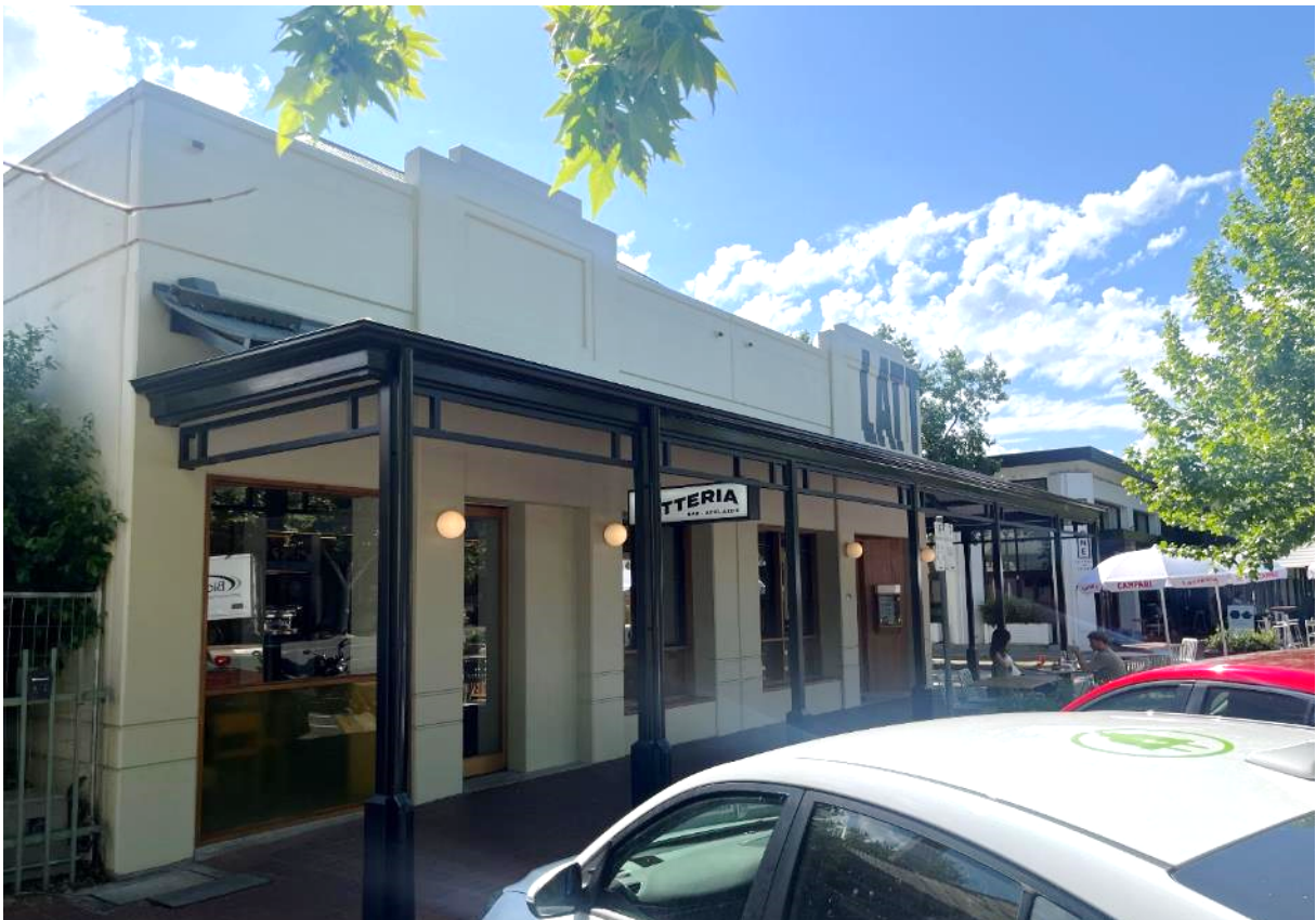
Figure 3.4 – View of neighbouring building to the north fronting Hutt Street
